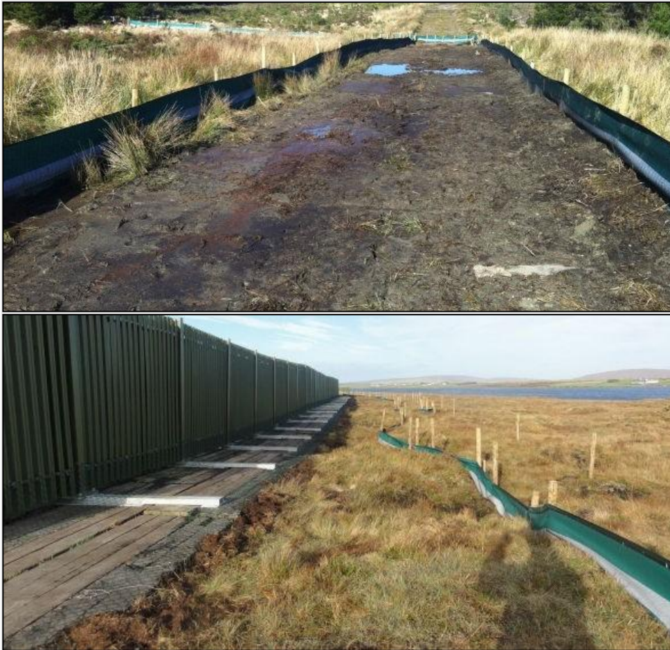
Plate 2-4: Typical Silt Fence Details
