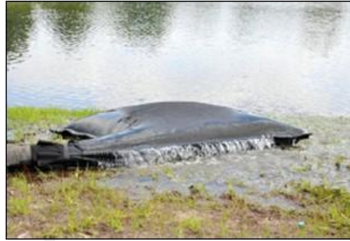
Plate 2-2 Silt bag with water being pumped through
