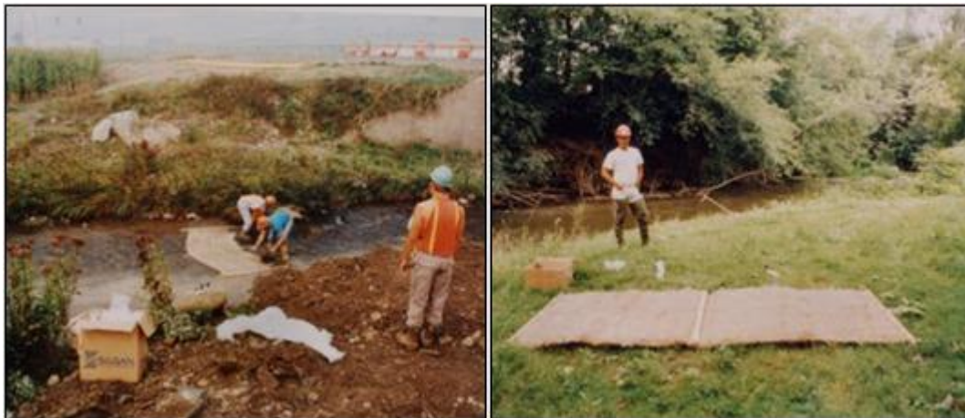
Plate 2-3: Typical Sedimat Details (Source: https://www.hy-tex.co.uk/ )
