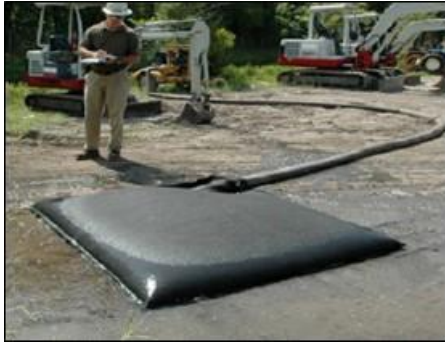
Plate 2-1 Silt bag under inspection
